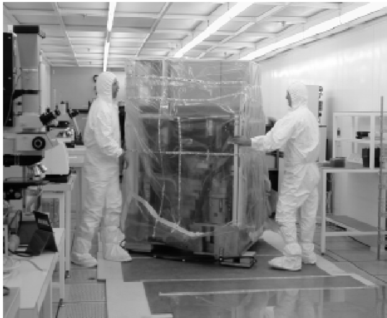
Figure 1. New equipment installation in the 150mm process line
